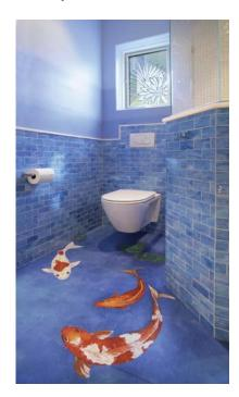
"The actuator plates are removable for maintenance access to the concealed tank and flushing mechanism. The plumber who installed it was particularly delighted at this," Giuliani points out. Installation of the carrier involved placing it within the studwork and then attaching it to the studs and floor – only four connections in all. The Geberit in-wall carriers have been tested to hold up to 880 lbs.
